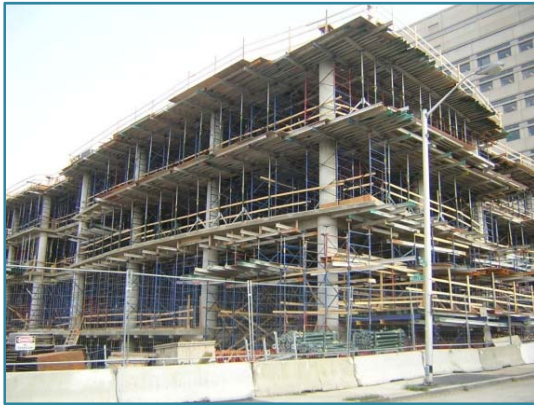
Current Cast in Place Structural Design
